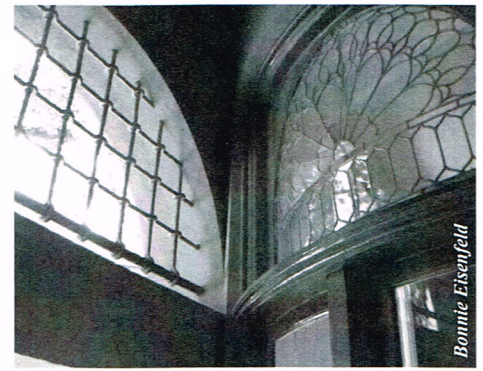
Architectural details feature a leaded glass fan light.
