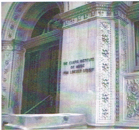
Curtis Institute of Music: 1726 Locust St. Originally the Drexel Mansion, built in 1894, notable for its Romanesque and Renaissance architectural details.
